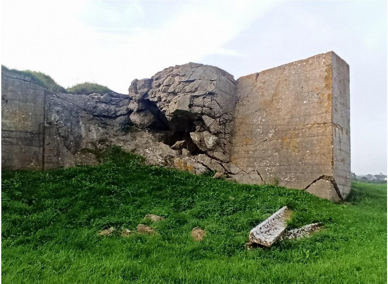
This is the exit hole in the back of Casemate #4 caused by the second projectile.
